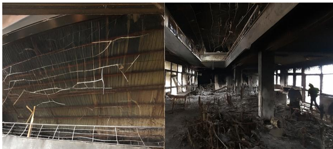
Fire Damage to CBE Building – Sheraro Branch (2022) The internal surfaces and roof of the Commercial Bank of Ethiopia (CBE) building in Sheraro sustained extensive fire damage, severely compromising structural integrity and service continuity. Source: CITG Survey (2022)
