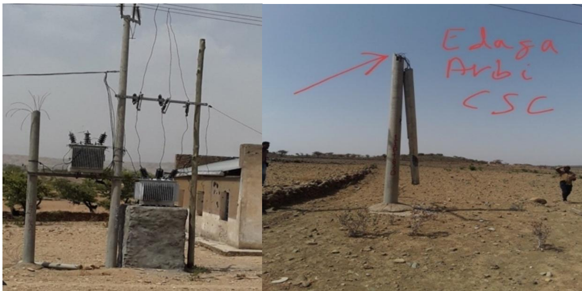
Figure 6-20: Destroyed Distribution Transformers and Concrete Poles at Edaga Arbi.
