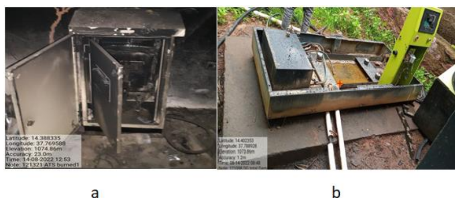
Figure 7-2: Damaged Diesel Generator(a) and Burnt ATS (b) at Sheraro Keramdi Ethio-Telecom Site
