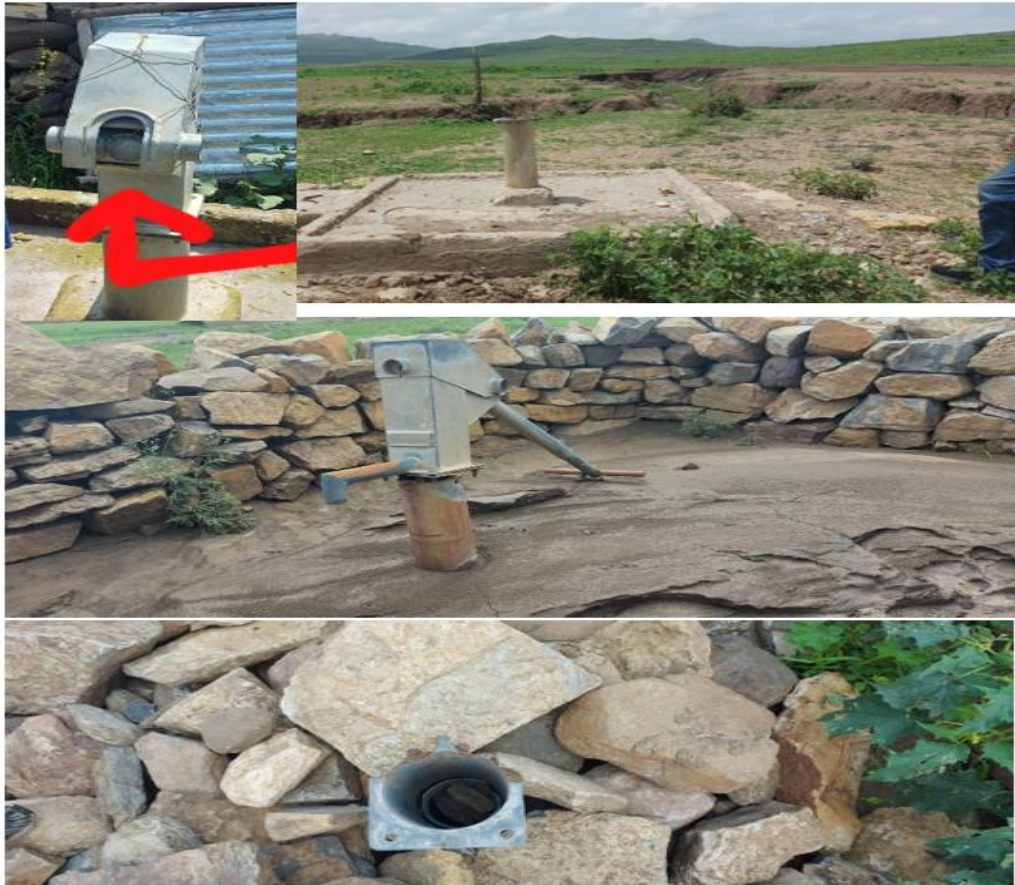
Figure 3-5: Damaged Hand Pump in a Rural Area
