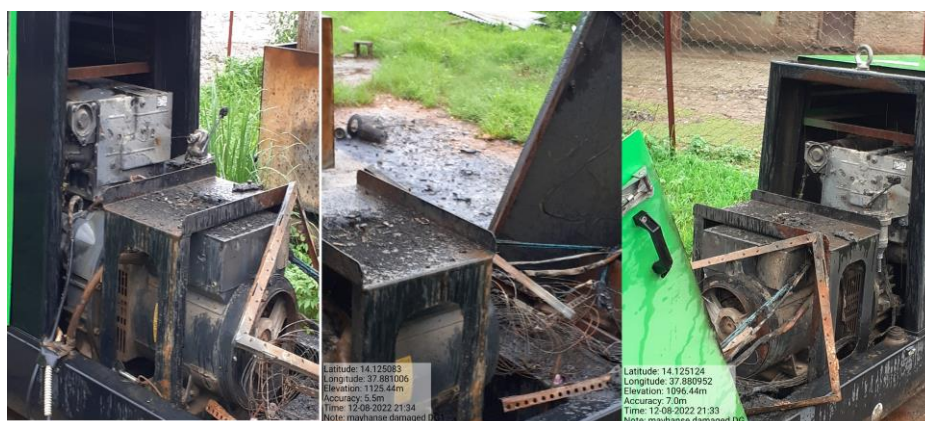
Figure 7-6: Burned Power Generator in May Hanse Ethio-Telecom Site
