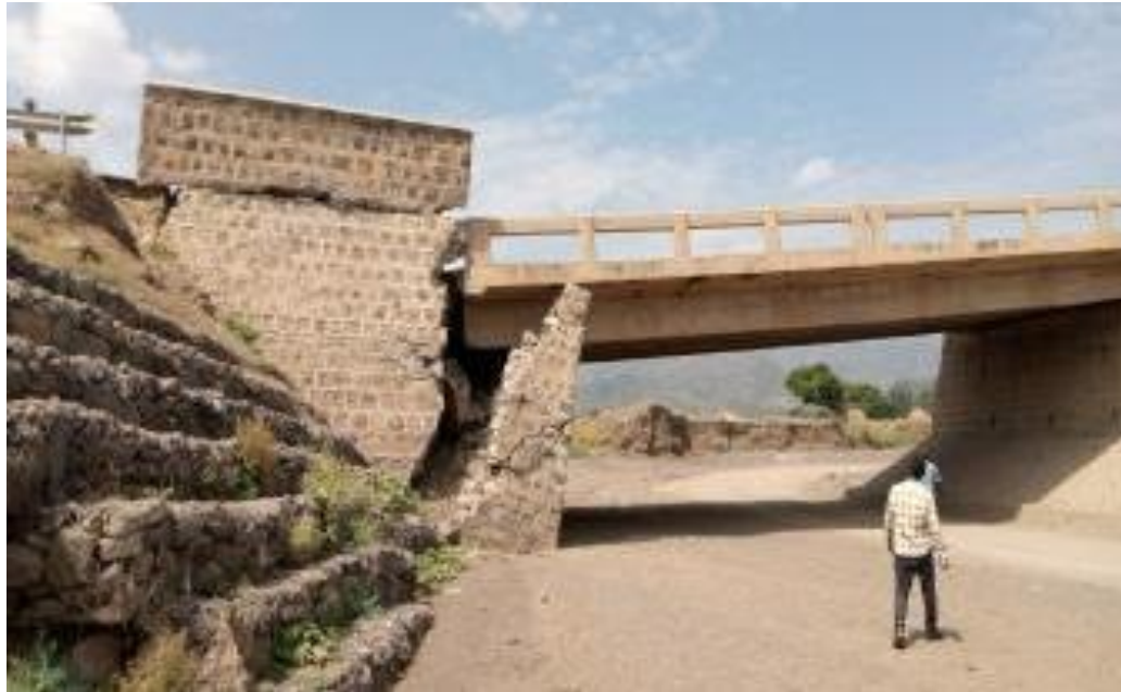
Figure 4-10: Garjale Bridge Damage (Alamata to Mekoni), Main Road from Amhara to Tigray (A bridge that was repeatedly loaded by many tanks and collapsed, Photo taken by TRA, November 2022), Source: CITG, 2022
