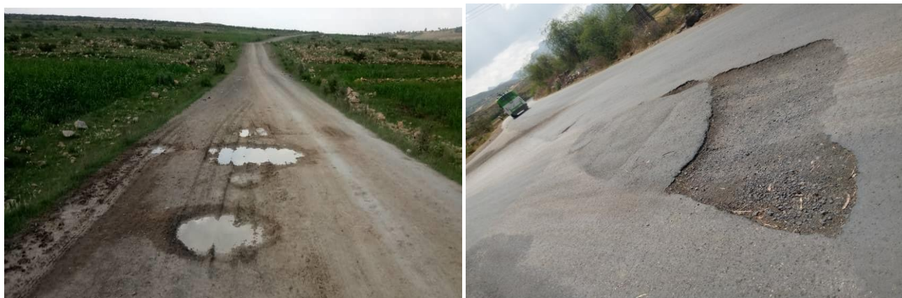
Figure 4-8: Sample Damaged Roads on Gravel and Asphalt Road Surface
