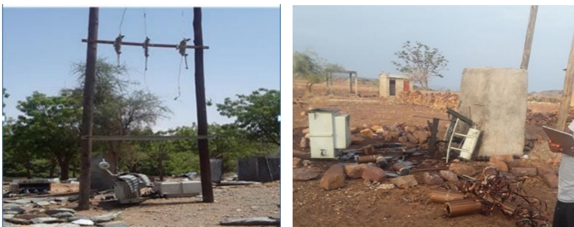
Figure 6-20: Destroyed Distribution Transformers and Concrete Poles at Edaga Arbi.
