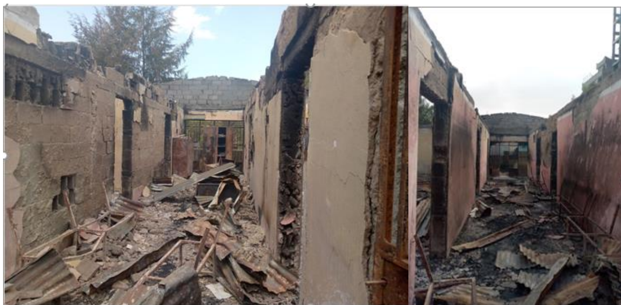
Figure 3-3: Damaged/Burned Water Supply Offices Building
