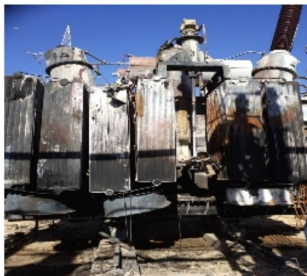
Figure 6-6: Destroyed 25MW Transformer at Tekeze Substation following Drone Strike
